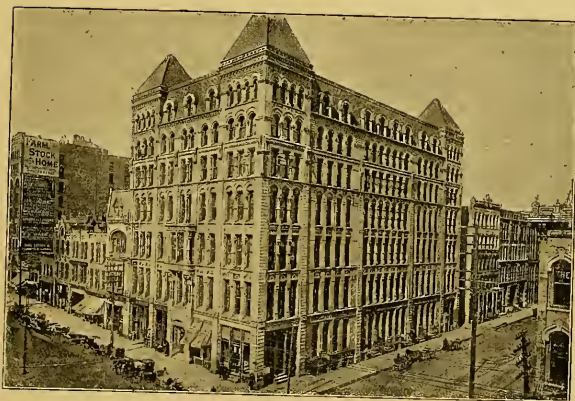
FIG. 128. THE BOSTON BLOCK, MINNEAPOLIS.
